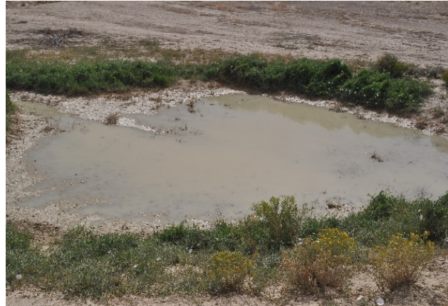
Figures 4 and 5. Diagram showing a conceptual diagram and image of a sediment/salinity retention pond near Delta, Colorado.
