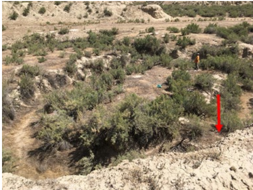
Figure 11. Photograph showing site 2 with the constructed berm (indicated by red arrow) on the downstream site.
